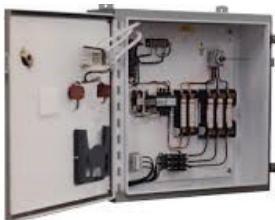
SCR Power Control & Contactor Relay Panels
